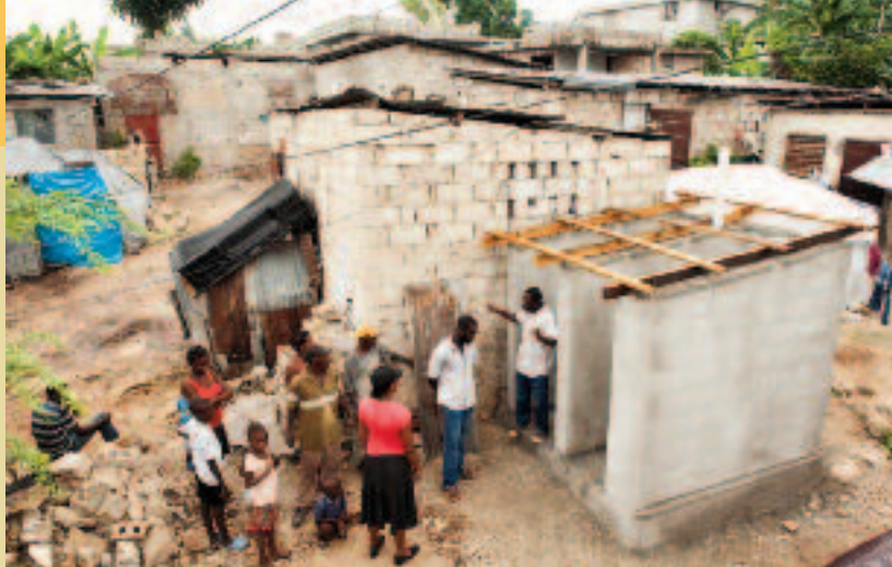
Building toilet facilities. Photo: © Éric St-Pierre/Oxfam Québec
